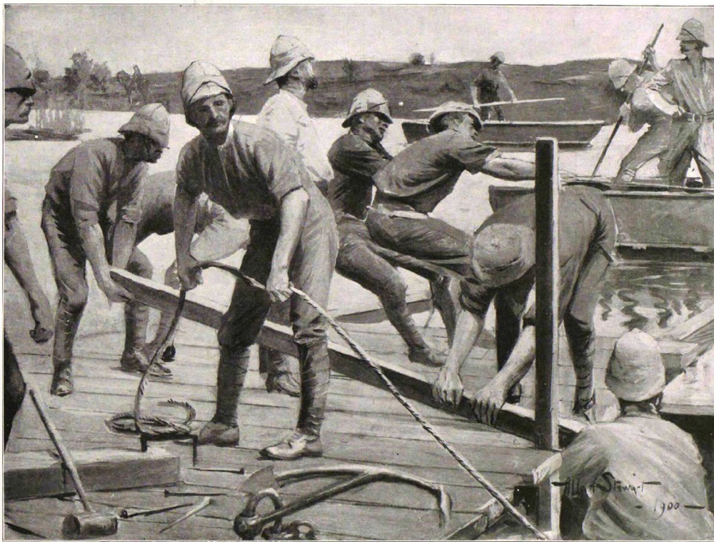
THE ROYAL ENGINEERS BUILDING A PONTOON BRIDGE OVER THE TUGELA.
